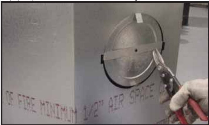
Figure 9.8 Cut the metal retaining band and fold the sides out.
