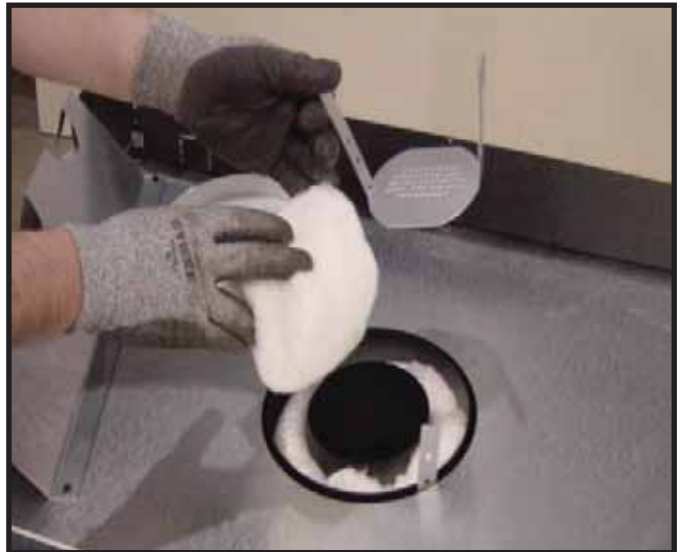
Figure 9.4 Remove the insulation basket and white insulation from the center vent pipe.
