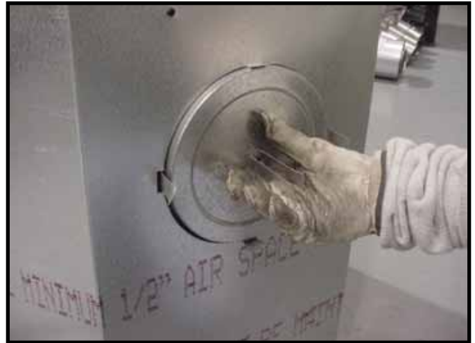
Figure 9.9 Fold the center parts of the retaining band out and use to remove the seal cap.
